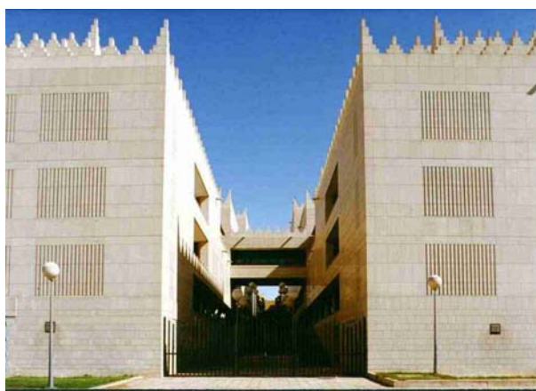
Figure5.3: Administrative buildings, design development by Beeah group, showing traditional facade character.
