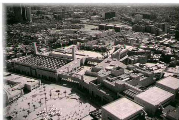
Figure 5.1: Aerial view of the Great Mosque of Riyadh, the Justice Palace and the three administrative buildings; on outgrowth of the Qasr Al-Hukum Study.
