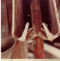
Close-up of one of the fourth floor beams.
