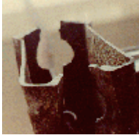
Underside view of one of the fourth floor beams.
