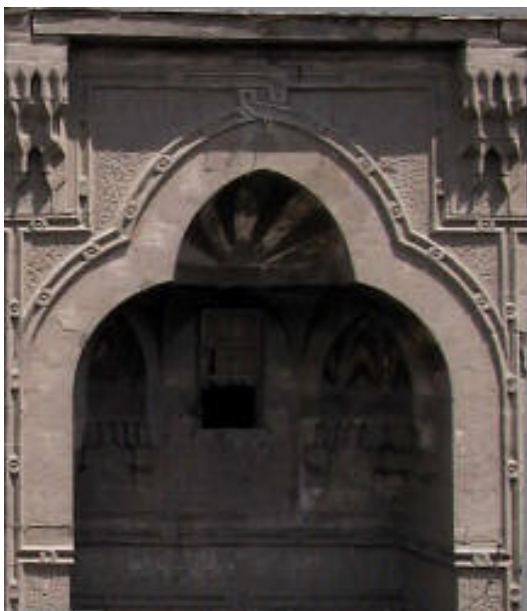
Figure 33 rectified image of the trifle formed arch in the top of the main entrance. (ECAE, 2005)
