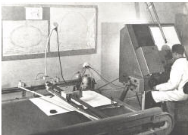
Figure 24 Analogue stereo pair photogrammetry; establishing a stereoscopic model in the bundesdenkmalamt (Vienna), the plotter is equipped with a 'calculator-corrector'; attached to the left of the operator's hand for inclined axis shots, and in turn it drives the mechanism on the drawing board. (UNESCO, 1972)
