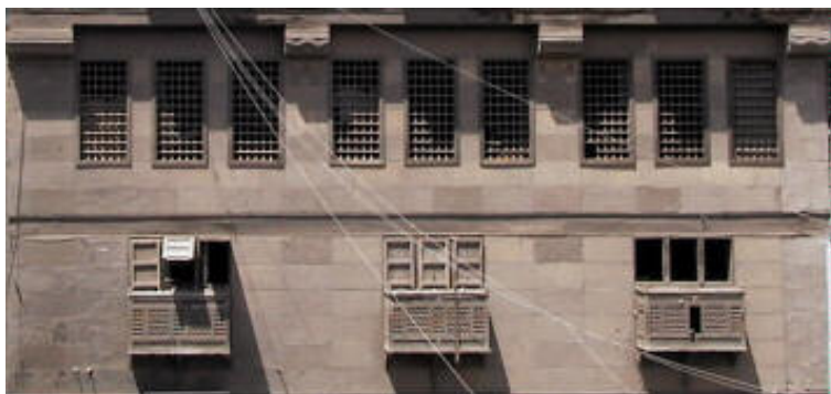
Figure 34 rectified elevation; using rectified elevation as a mapping material for the production of the textured model. (ECAE, 2005)
