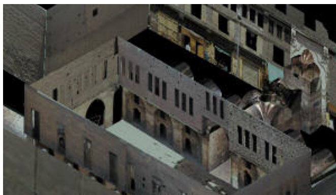
Figure 38 3D reconstruction isometric view of the building; Obtaining a model within a reasonable time, then details can be fulfilled later to complete the project (ECAE, 2005)
