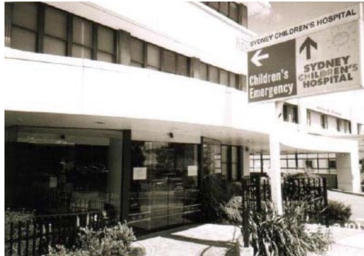
An emergency department attached to a large teaching hospital.
