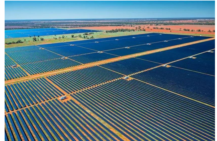
Sudair Solar PV Parks
