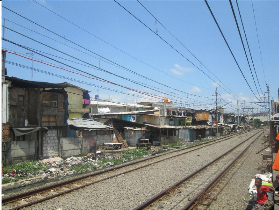
Figure 3. Unstable location of Kampung Bandan & Muko. The residents of these settlements take advantage of the areas adjacent to the railway line to build their housing, which does not comply with the building regulations. I noticed during my visit to this kampung that children are playing in the train track area. Fortunately, the train reduces speed when passing through this area! Source: Author.
