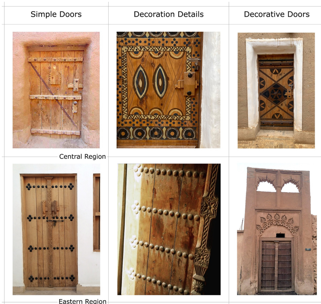
Fig. 8. The various details and richness of wooden doors in the central and eastern regions of Saudi Arabia.
