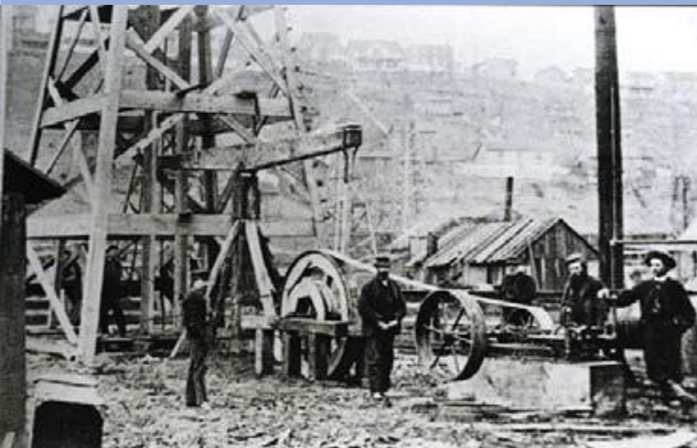
■ Typical Percussion Cable Rig
