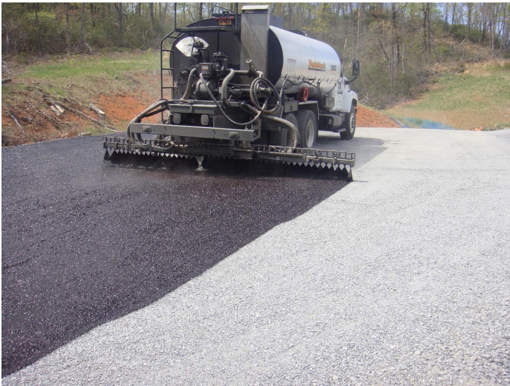
Figure 4: fog seal.
