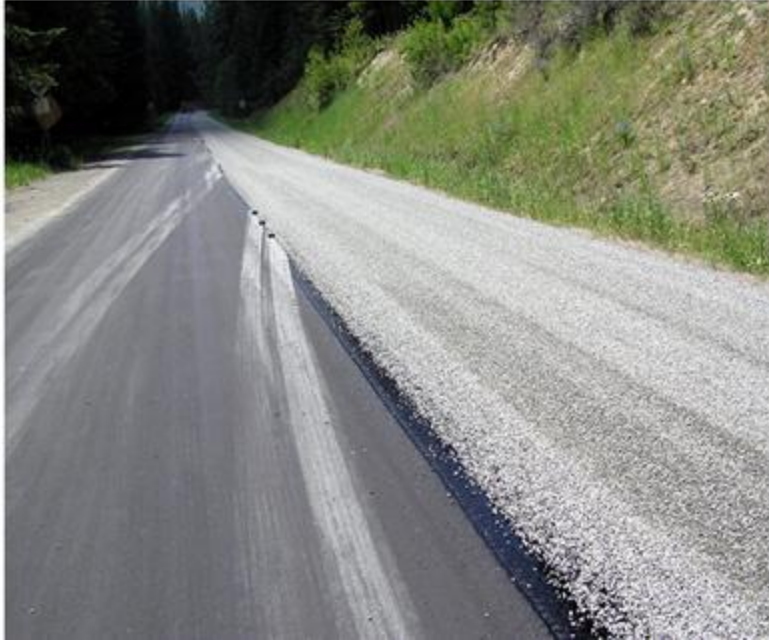
Figure 7: Chip seal rehabilitation over a BST.
