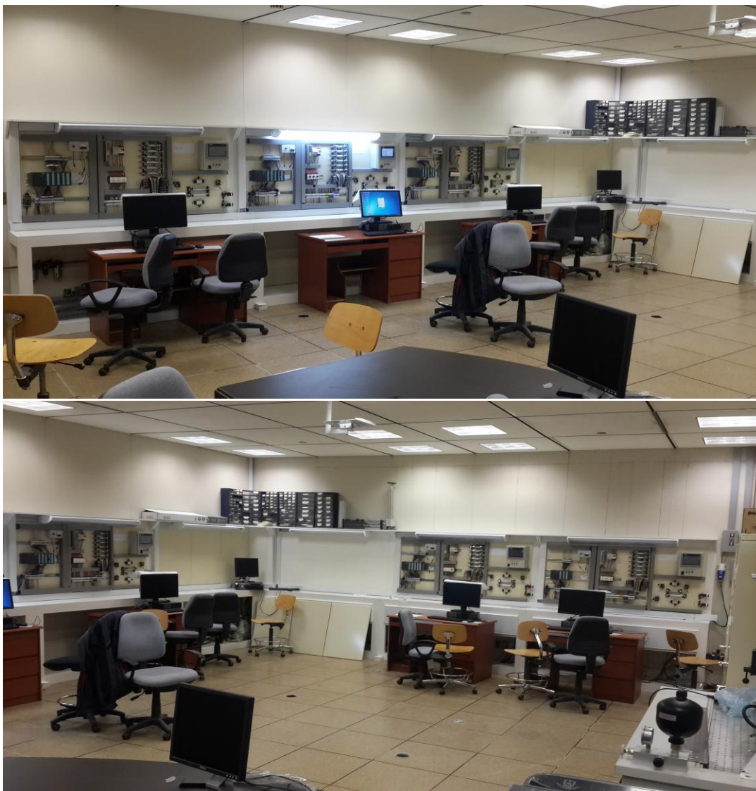
Figure 2.1 S7-300 PLC training stations at Industrial Engineering depart automation laboratory.
