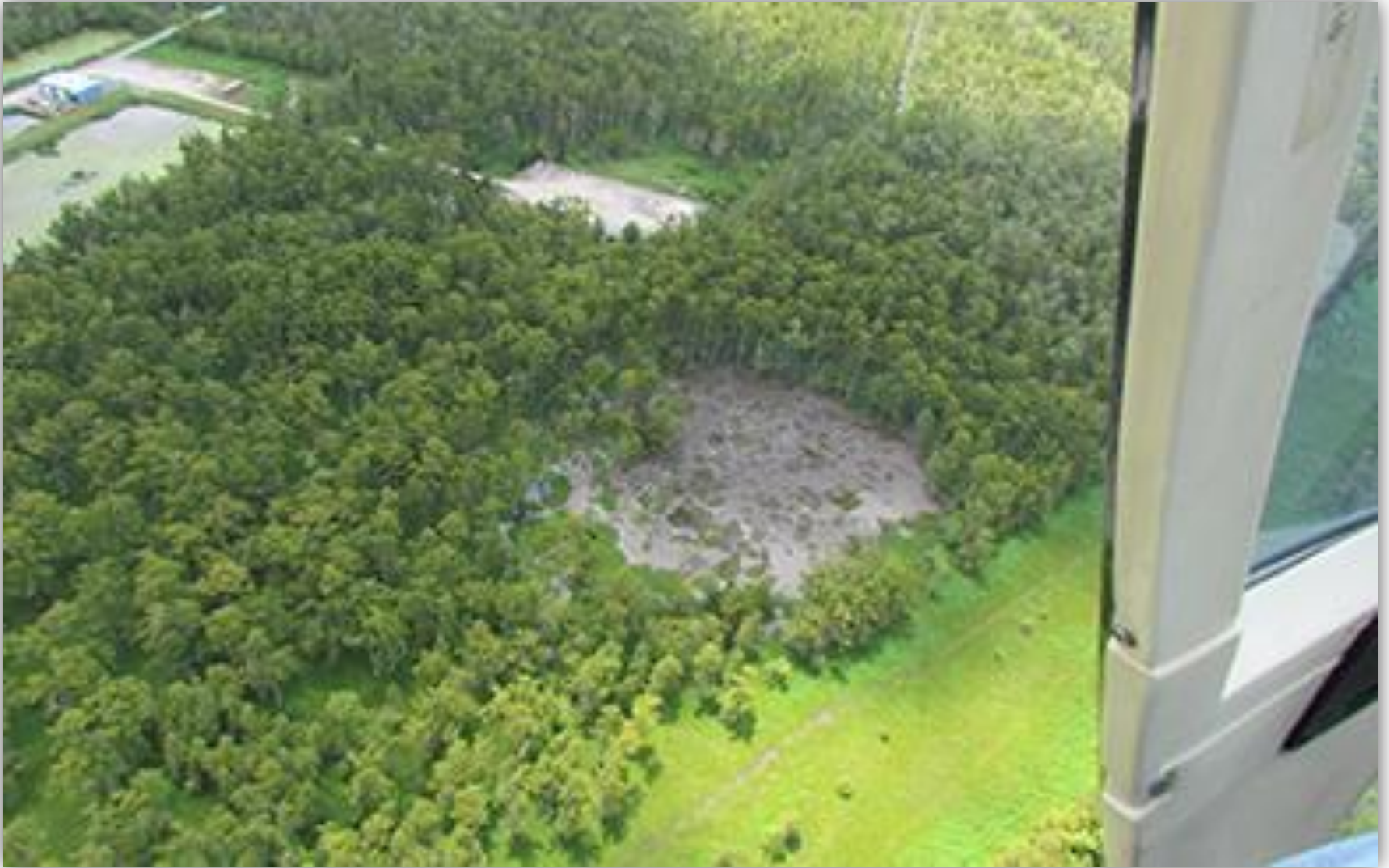
Aerial Photograph taken for a site – shows a possible sinkhole
