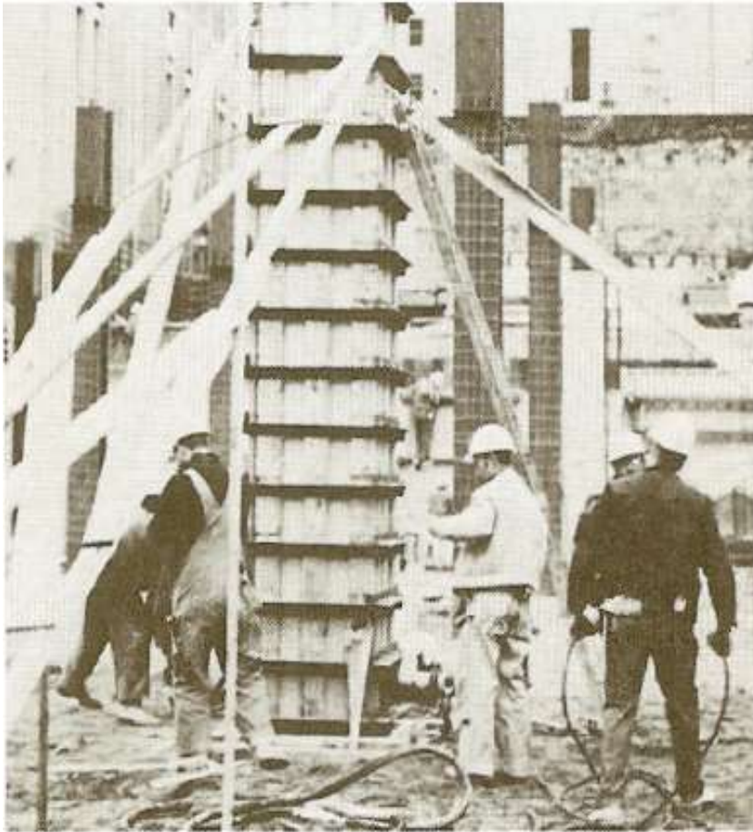
FIGURE 12-3: Pumping concrete into bottom of column form. (Courtesy of Gates & Sons, Inc.)
