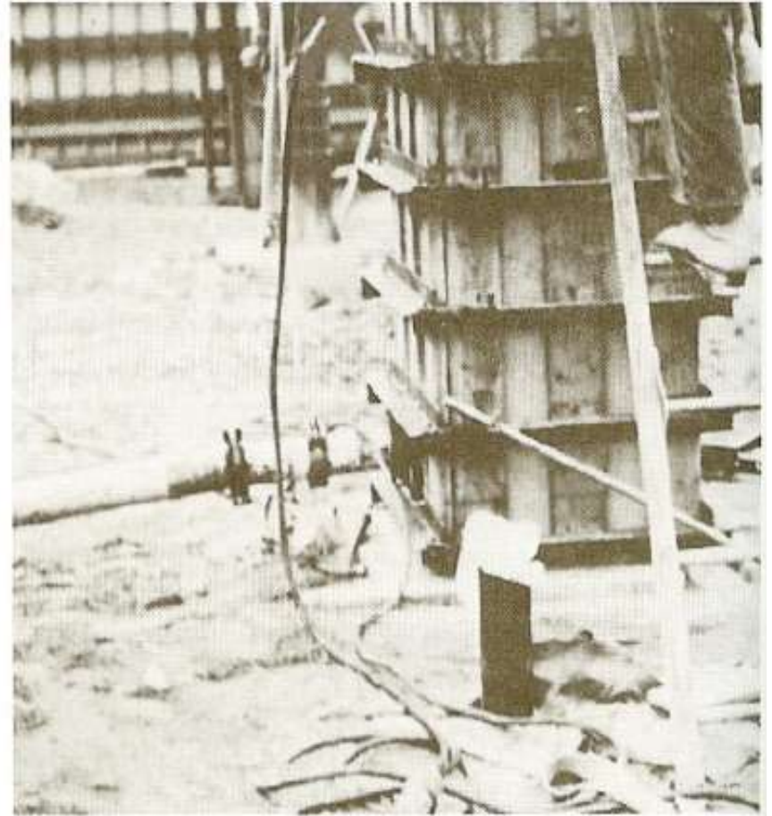
FIGURE 12-3: Pumping concrete into bottom of column form. (Courtesy of Gates & Sons, Inc.)
