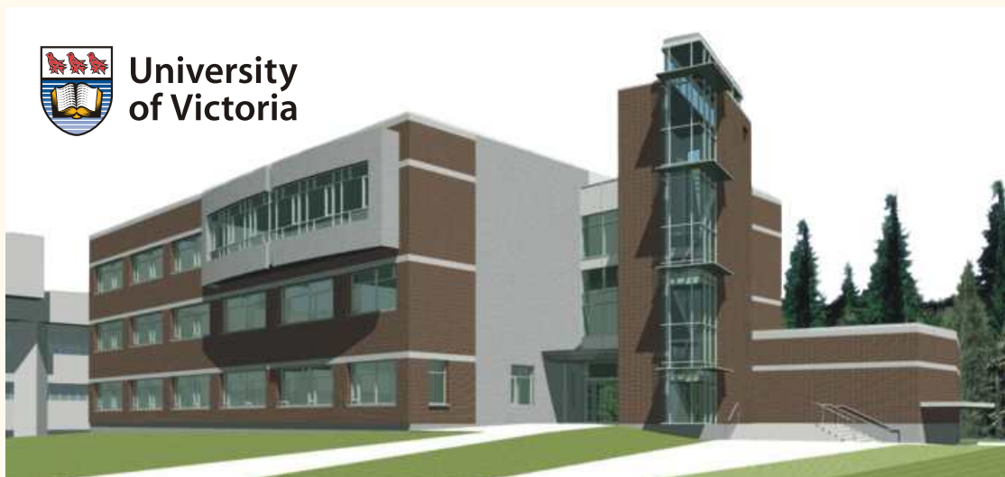
Island Medical Program Building
