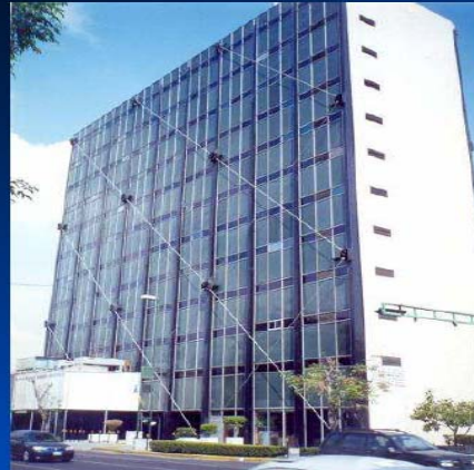
Cable bracing for 12-story steel frame
