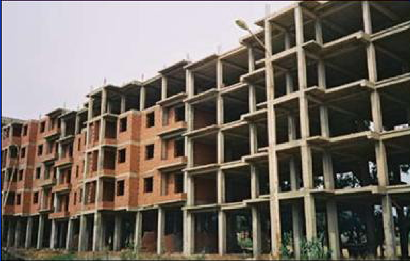
5-story and multi-bay Reinforced Concrete Frame Structure
