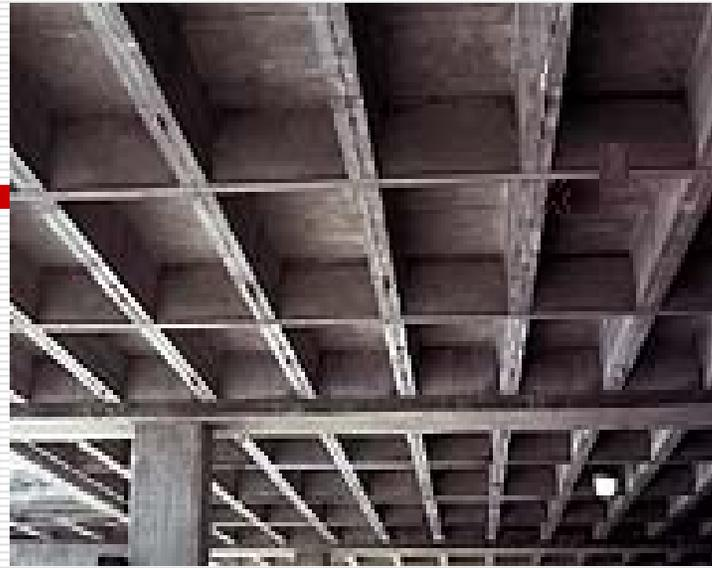
**Image-GoddenF76** Typical one-way beam grid and slab system. This parking structure has columns on a rectangular grid pattern. The essentially one-way design of the system can be seen by the relative lengths and sections of the main beam, and the primary and secondary beams under the slab. The rectangular shape of the unsupported slab also indicates one-way slab action.
