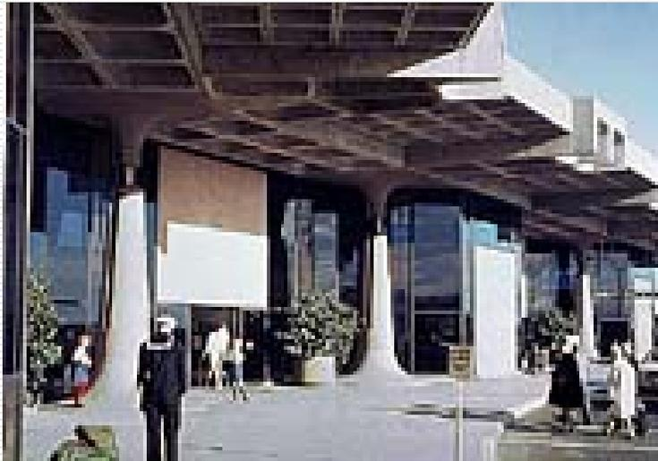
[Image-GoddenF78](#) Waffle-slab roof, San Diego Airport. Not heavily loaded as a roof structure, the waffle slab system could be extended into the overhang where the moments are negative. Note also the supporting columns with a built-in point of zero moment at two-thirds height. (San Diego, California)
