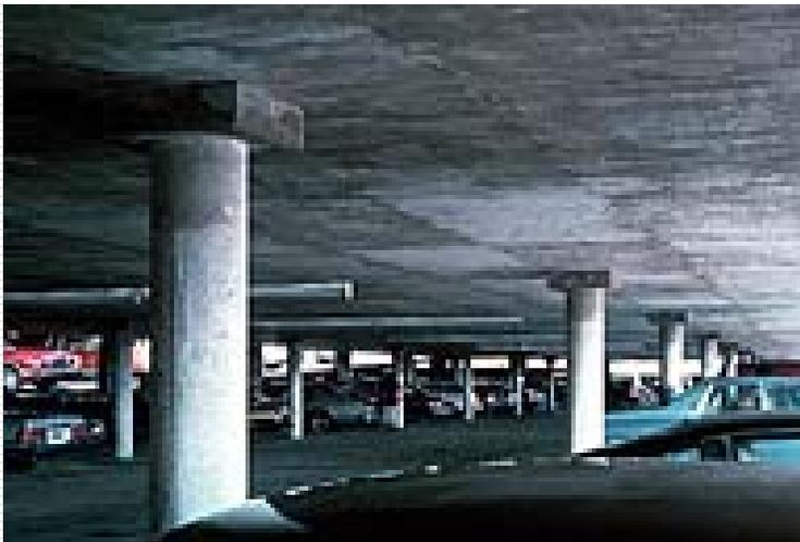
[Image-GoddenF79](#) Typical flat slab construction for a parking structure. Note the square column capitals that increase the area of the slab resisting punching shear at the columns.
