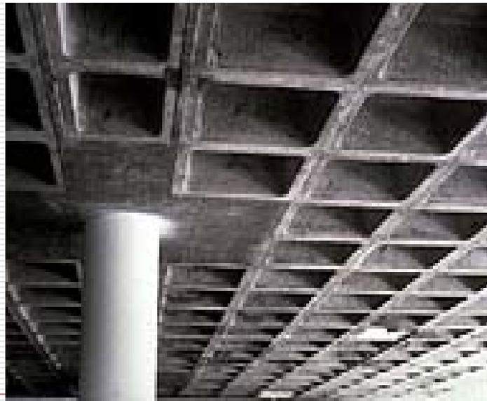
**Image-GoddenF77** Typical waffle-slab for parking structure. With columns on a 33-ft x 27-ft pattern, the design uses 3-ft square waffles. Note the infilling of the squares at the head of the column to resist both shear and negative moments.
