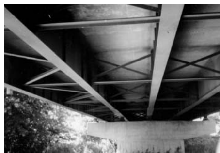
Figure 3 Composite plate girder bridge with X-shaped diaphragms.
